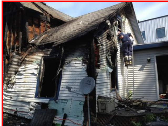
Explosion and resulting fire caused by extracting hash oil using butane.
